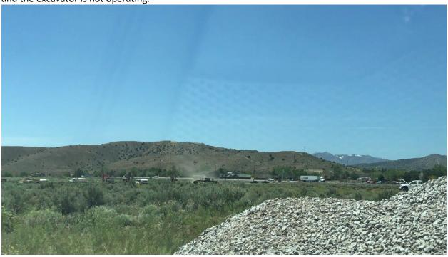
Photograph 2 Date: 05/24/2022 Direction: Southwest Image demonstrates uncontrolled fugitive dust from a blade and excavator operating at the Stonebrook Apartments project site without dust mitigation. Note the parked Aspen Earthworks water truck between the blade and the excavator is not operating.
