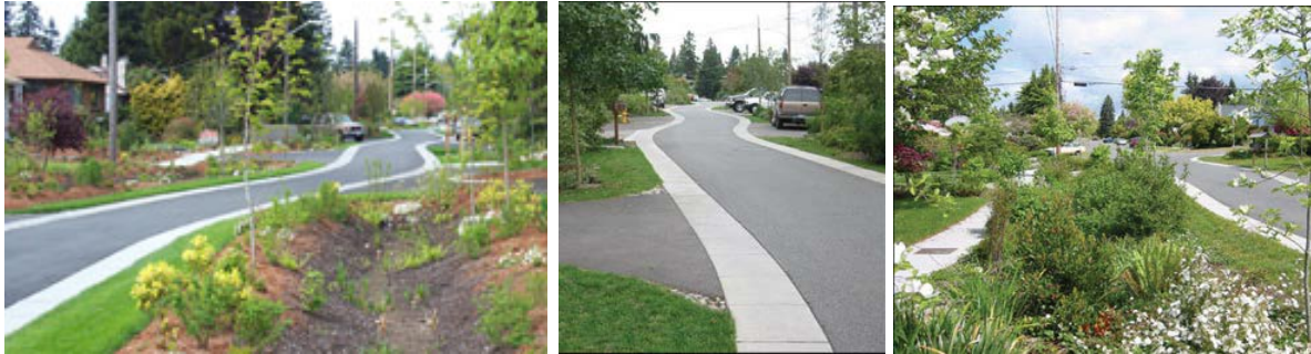
Figure 4-6. Images of SEA Project streets (images courtesy of Seattle Public Utilities District)
