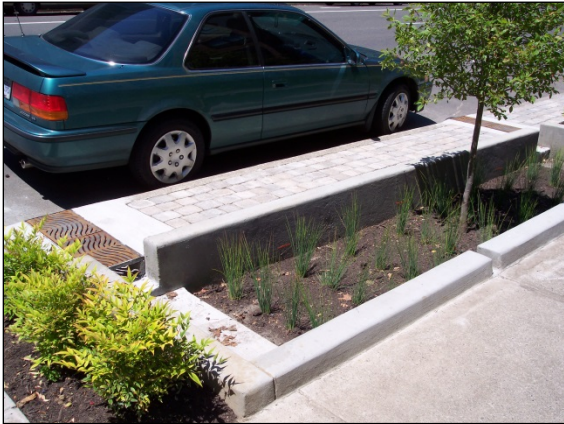
Figure 4-13. Street-side bioretention.
