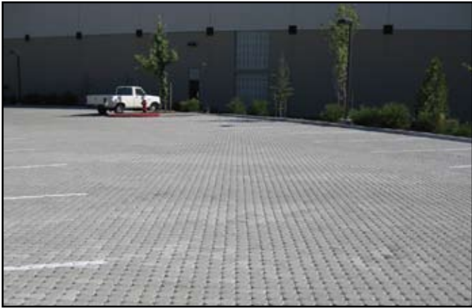
Porous pavement was installed in this commercial parking lot.
