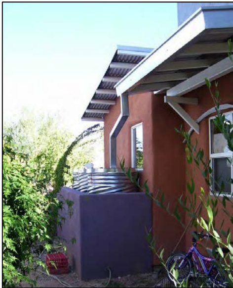
Figure 4-24. A rainwater catchment system on a residential home. (Source: Kennedy/Jenks Consultants)
