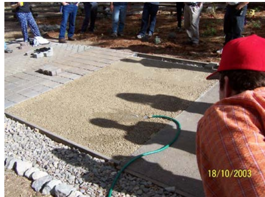
Figure 4-20. Demonstration project at Lake Tahoe. Underlying clean gravels being installed (left) and water rapidly infiltrating into porous concrete (right).
