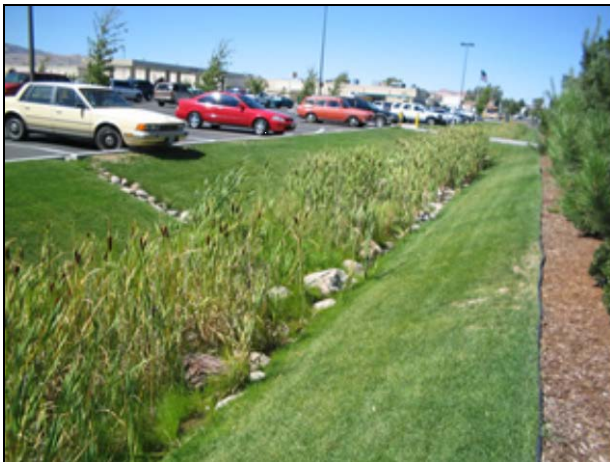
Figure 4-2. Parking lot bioretention.
