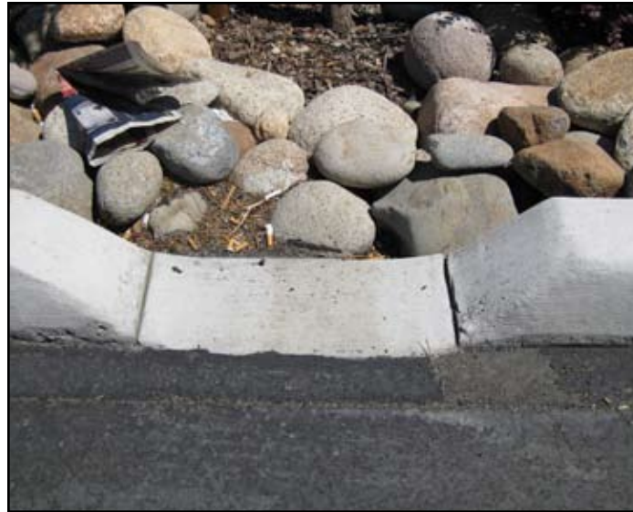
Routine maintenance of this parking lot inlet consists of sediment and trash removal.
