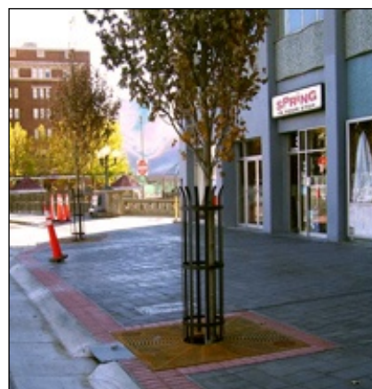
Figure 4-12. Tree box filter installed in downtown Reno.
