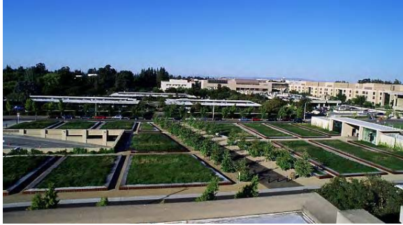
Figure 5-3. Intensive Green Roof on a parking structure at Stanford University, Palo Alto, California. (Source: Rana Creek)
