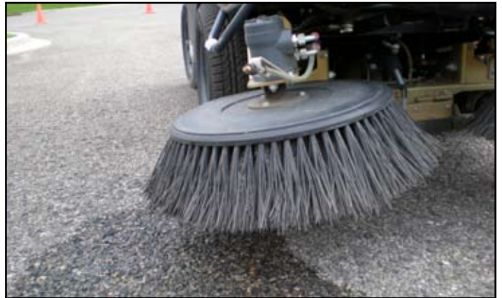
Routine maintenance of porous pavement includes vacuum sweeping at least twice a year.
