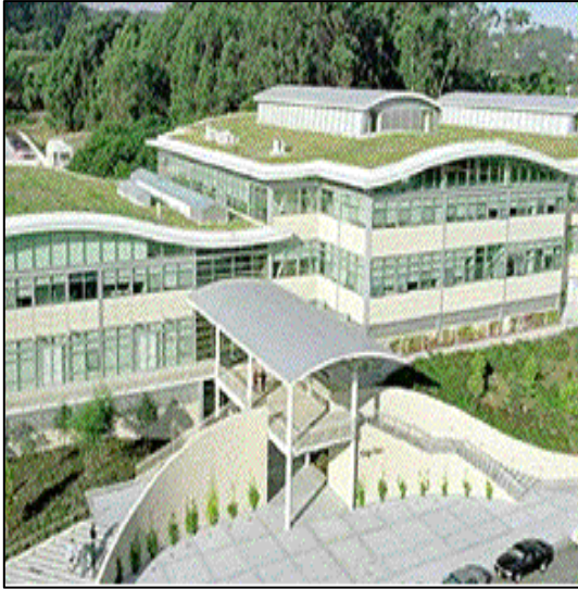
Figure 4-26. Green Roof at GAP Corporate Campus, San Bruno, CA. (Source: Rana Creek)
