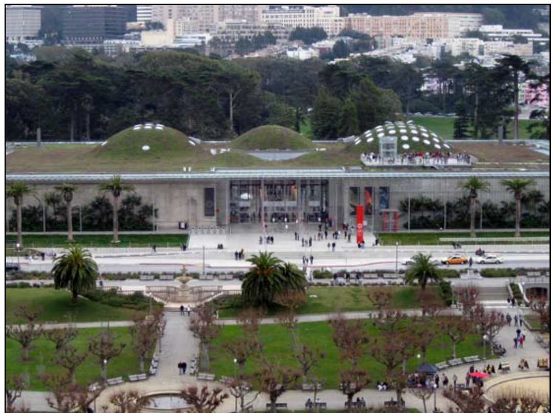
This green roof in San Francisco provides a way to capture and infiltrate rain water, reduce stormwater runoff and augment valuable green space.
