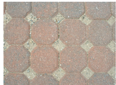
Figure 4-23. Brick pavers. (Source: NEMO Nevada)
