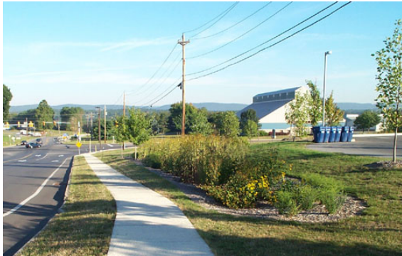
Figure 4-8. This sidewalk at Pennsylvania State University is made of porous concrete. (Photo courtesy of Cahill Associates )
