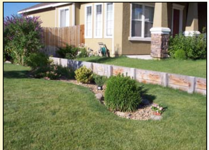
This residential rain garden captures and filters runoff water.
