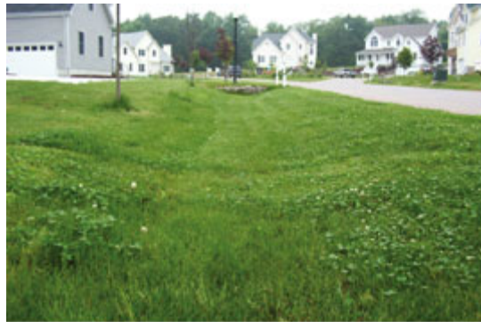
Figure 4-5. An uncurbed road utilizing a vegetated swale.
