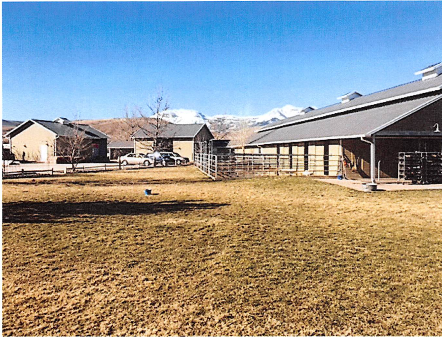
Photo of Existing Stables
