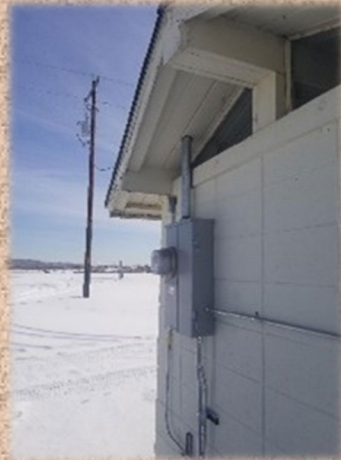
Remodel of bathrooms on holes 2 and 17. $90,000
