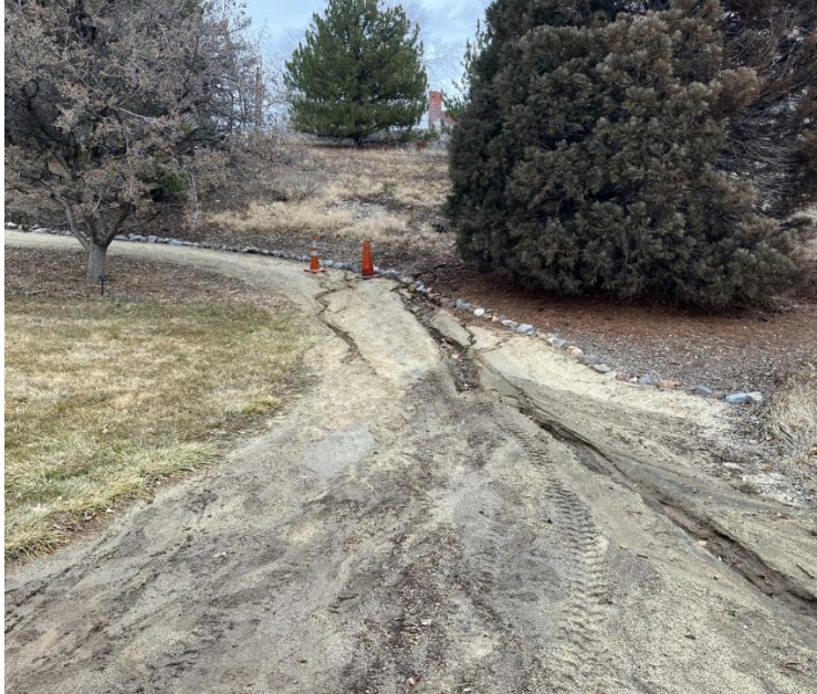
Trail repair: Before / After
