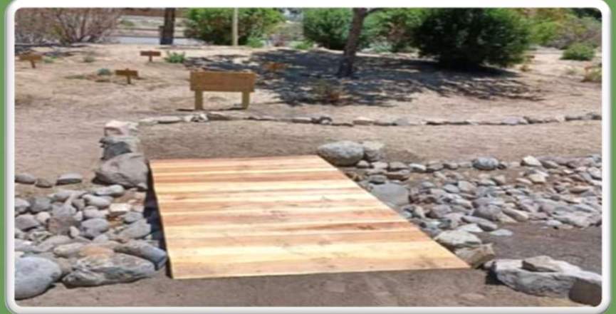
After photos of new bridge.
