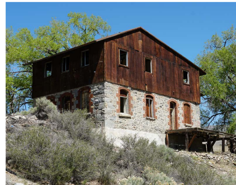
Avansino Ranch House
